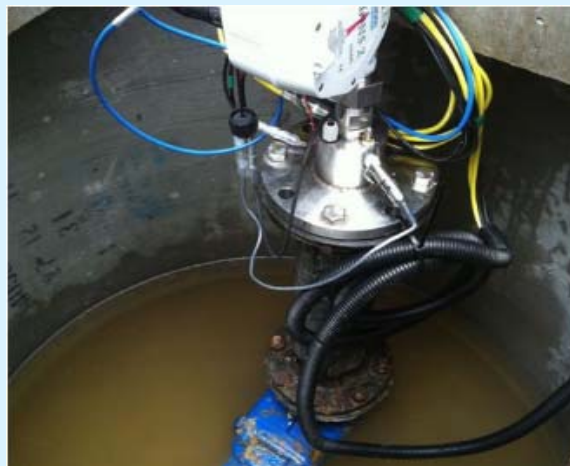
Figure 30 – WaterWiSe multi parameter sensor attached to a gate valve
