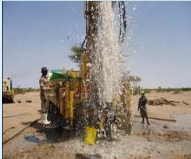
Figure 20 – Water gushing out of a Napuu area borehole
